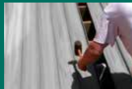
Lay Down Deck Board
