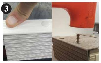
Place each Push Pin against the 1/4" pre-drilled hole. GENTLY push in with your thumb or tap the Push Pin into place using a non-maring mallot until it is level (flush) with the Gorilla Deck Trim.
